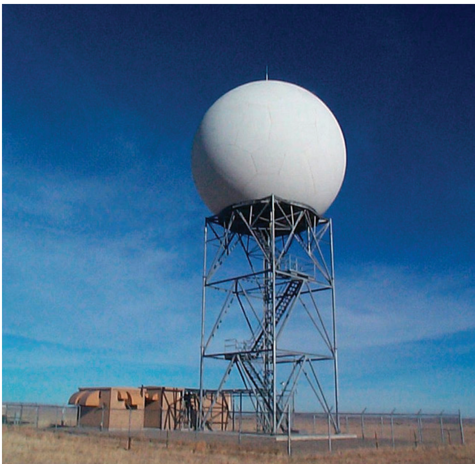
FIGURE 2.7 Photograph of a WSR-88D radar (NEXRAD) operated by the U.S. National Weather Service. SOURCE: NOAA.
