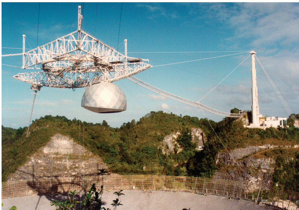
FIGURE 6.1 ( Left ) the 305 m NSF Arecibo antenna. The 2.38 GHz transmitter is housed in the dome, while the 430 MHz transmitter is in the operations building with the power being delivered to the line feed to the left of the dome via a waveguide coming up the catwalk from the base of the tower in the image. ( Right ) The 70 m NASA Goldstone DSN-14 antenna. SOURCE: ( Left ) Courtesy of NAIC/Arecibo Observatory, a facility of the NSF. ( Right ) Courtesy of NASA/JPL.
