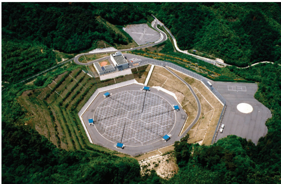
FIGURE 2.8 The MU radar in Shigaraki, Japan. This example of an MST radar has an antenna field with an overall aperture diameter of approximately 100 m. SOURCE: Hiroyuki Hashiguchi, Kyoto University.
