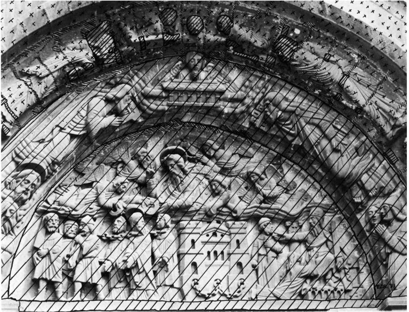
Fig. 15. Saint-Denis, west facade, left portal, diagram of restorations to the tympanum and archivolt
