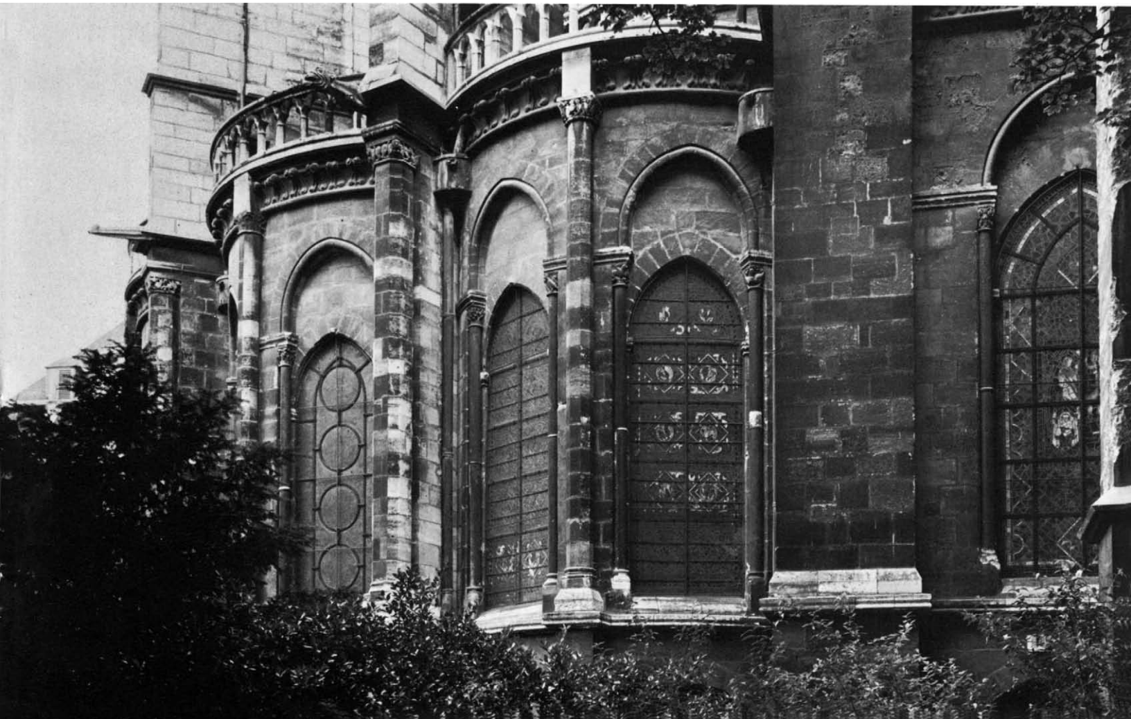
Fig. 9. Saint-Denis, upper windows of the chevet, north side
