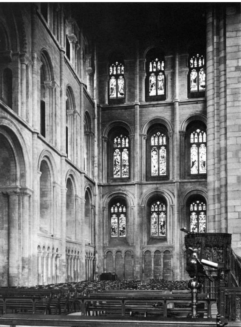
Fig. 1. Peterborough Cathedral, interior of north transept
