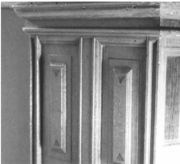
11. Detail of the side of figure 10, showing double-fielded panels and a broad sunken band on the upright
