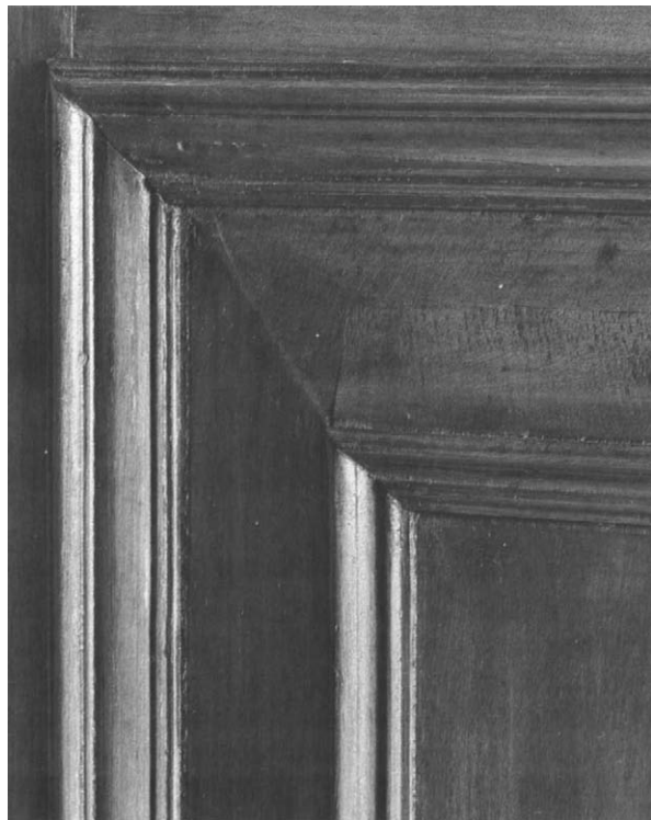
40. Detail of door of catalogue number 11. Note the patch inset in the top bevel of the panel, replacing wood removed when the central field was plowed out with a plane. (See fig. 24, b.)
