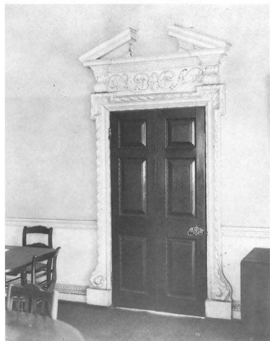
FIGURE 16. Doorframe , 1772-73, dining room, the Chase-Lloyd house, Annapolis. Photograph, ca. 1900
