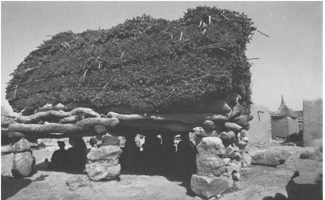
Fig. 1 Made of thickly stacked millet stalks, the roof of a men's meeting house, togu na , keeps the interior dark and cool. In this togu na the roof is supported by stone pillars rather than by carved wooden support posts (see nos. 41 and 42). Photograph by Eliot Elisofon, Ogot du Haut, January 1971; courtesy of National Museum of African Art, Eliot Elisofon Archives, Smithsonian Institution.
