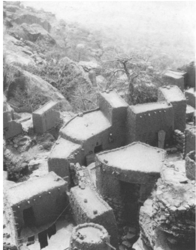
Fig. 4 Because of the shortage of flat land available for construction on the Bandiagara cliffs, the rooms of a Dogon compound are irregular in shape and arrangement and staggered in height. Photograph by Arthur Tress, 1967.
