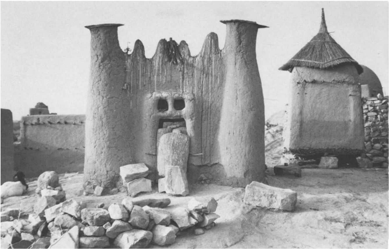
Fig. 8 Binu sanctuaries are identified by the turrets and mounds that rise from their facades. In this example an iron gobo hook has been inserted next to the turret on the left, and several domolo staffs are stacked in the center above the door. Sacrifices of blood and millet porridge have dripped down the front of the building. Photograph by Eliot Elisofon, Ogot du Haut, March 1972; courtesy of National Museum of African Art, Eliot Elisofon Archives, Smithsonian Institution.
