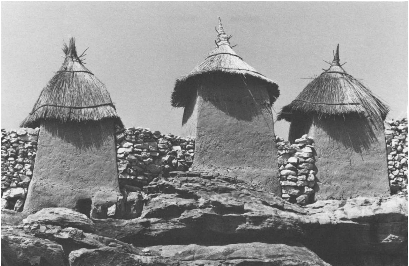
Fig. 6 These three thatched-roofed, mud-brick granaries are connected by a stone wall. Granaries hold reserves of food from one harvest to the next. Photograph by Lester Wunderman.
