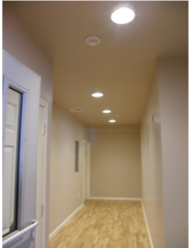
FIGURE 5.7 Example of downlighting. Sea Gull Lighting/Juice-Works. SOURCE: Next Generation Luminaires, PNNL.
