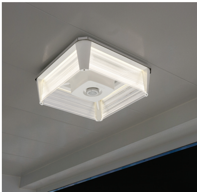
FIGURE 4.1 Cree IG Series WaveMax. The luminaire uses optical waveguides to provide low-glare illumination. SOURCE: Cree, “LED Parking Structure: IG Series Outdoor Lighting,” http://lighting.cree.com/products/outdoor/parking-structure/ig-series , accessed August 9, 2016.
