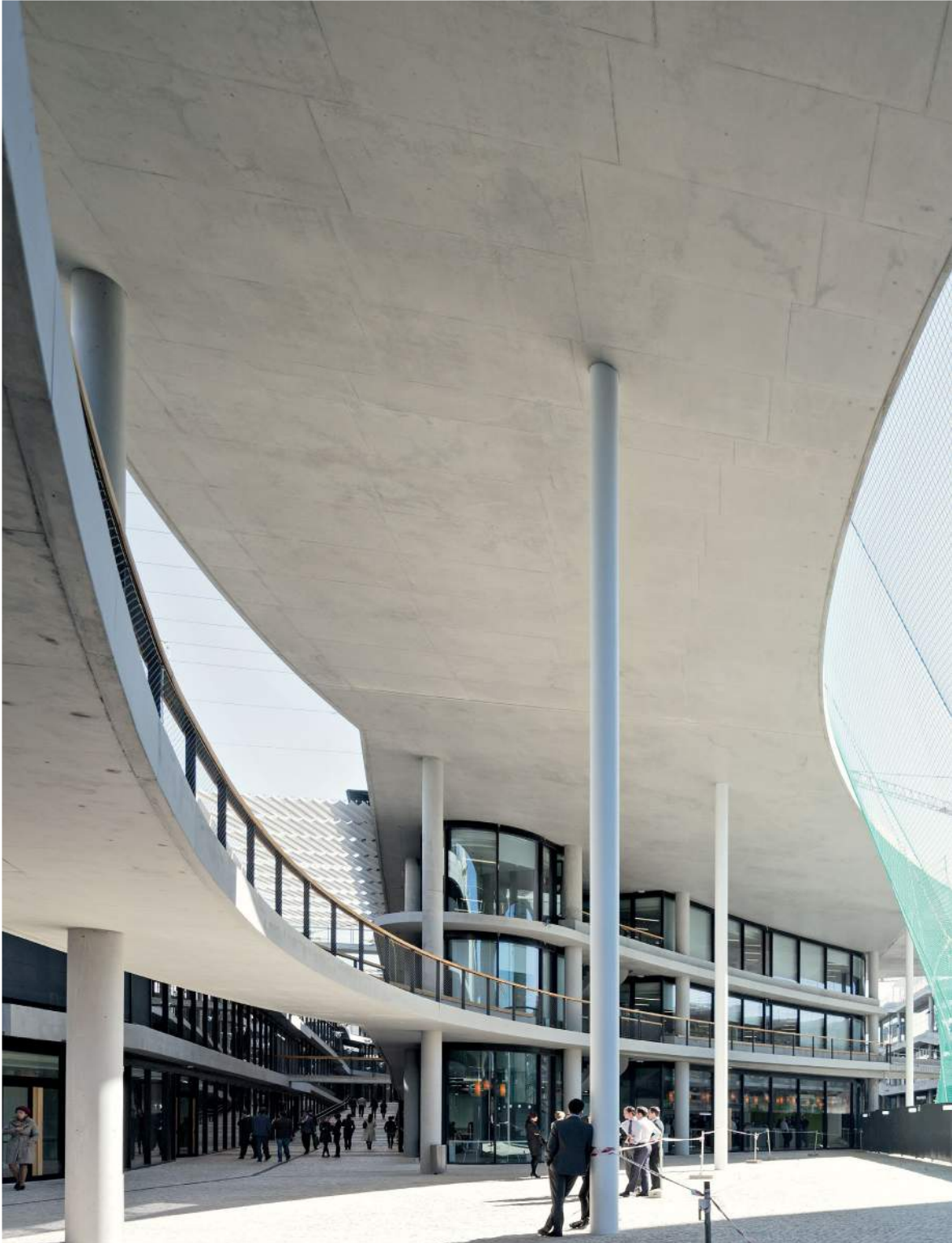
At the Plaza, the «Old» and the «New» town come together. The shape of the Plaza echoes that of the high-rise
