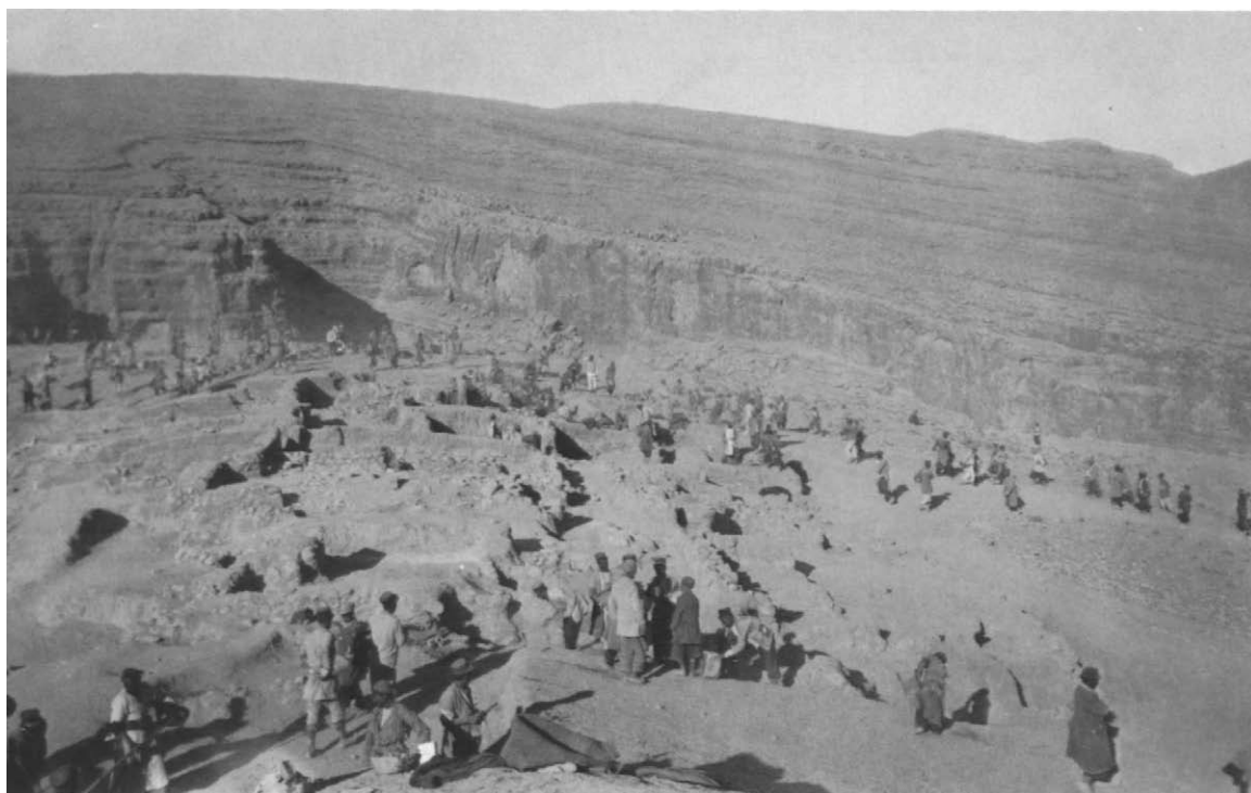
top: PL. 29. View of the fortress from southwest, second defense in the foreground bottom: PL. 30. Excavations in progress, from the podium looking north
