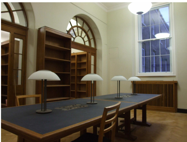
Refurbished small reading room ■ Room 182 A
