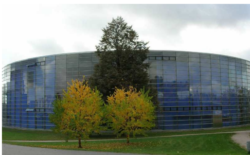
Facade (Photo: Jari Laine)
