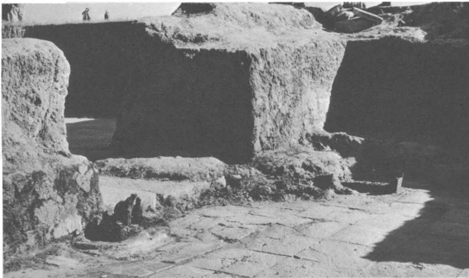
FIG. 3 The remains of the base of Assurnasirpal gates in situ. Temple of Mamu, Balawat.
