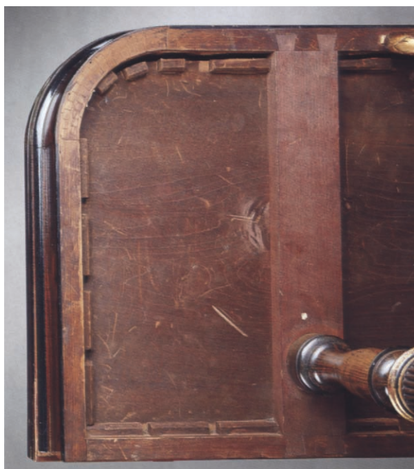
PLATE 96. Detail of the underside of the card table by a New York maker, plate 45, showing the use of glue blocks rather than nails to secure the bottom boards to the frame
