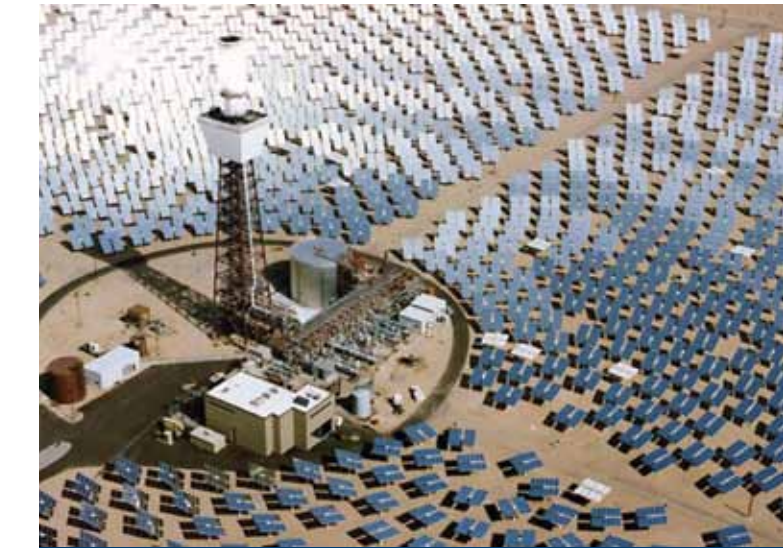
Technology first developed in the mid-1990s at projects such as Solar Two (above) in the Mojave Desert demonstrated that solar heat stored in thermal towers could be used to produce steam to power turbines to generate electricity.
