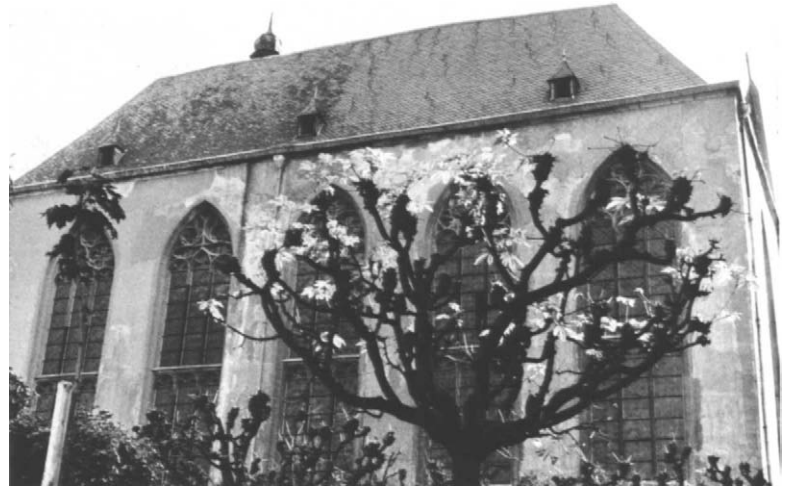
93 The north wall of the north nave of the Carmelite church at Boppard-am-Rhein
