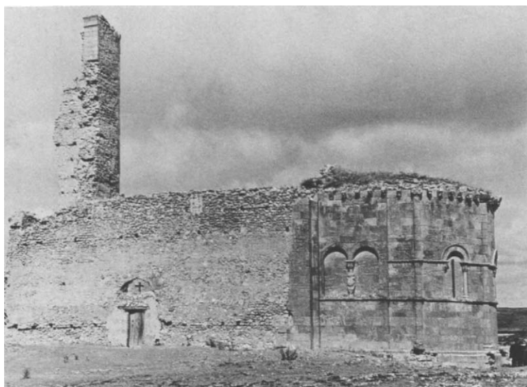
42 The exterior of the church of San Martín de Fuentidueña in 1955 before the removal of the apse
