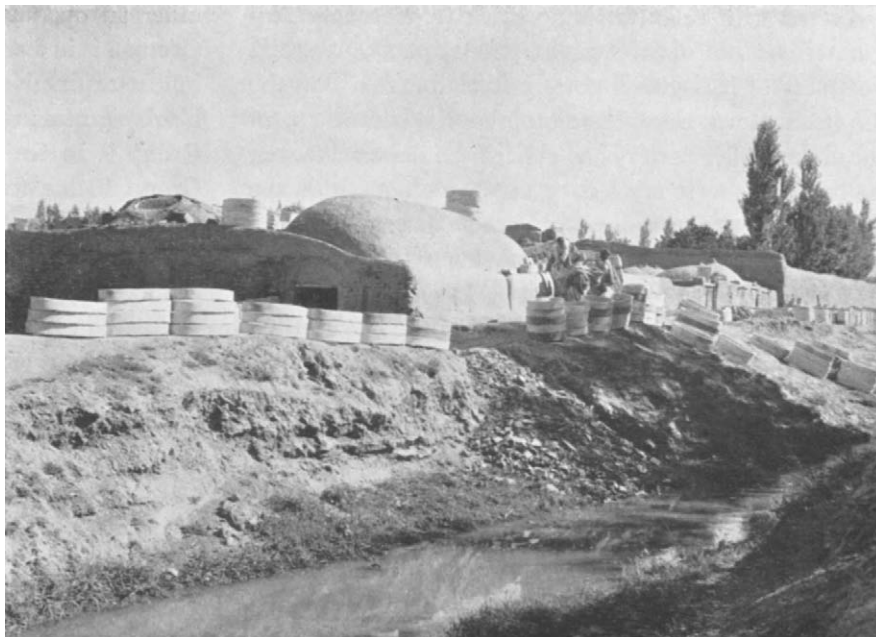
FIGURE 19 The largest kiln, with a shaftway in its ledge. Above the lower opening is evidence of brick patching.
