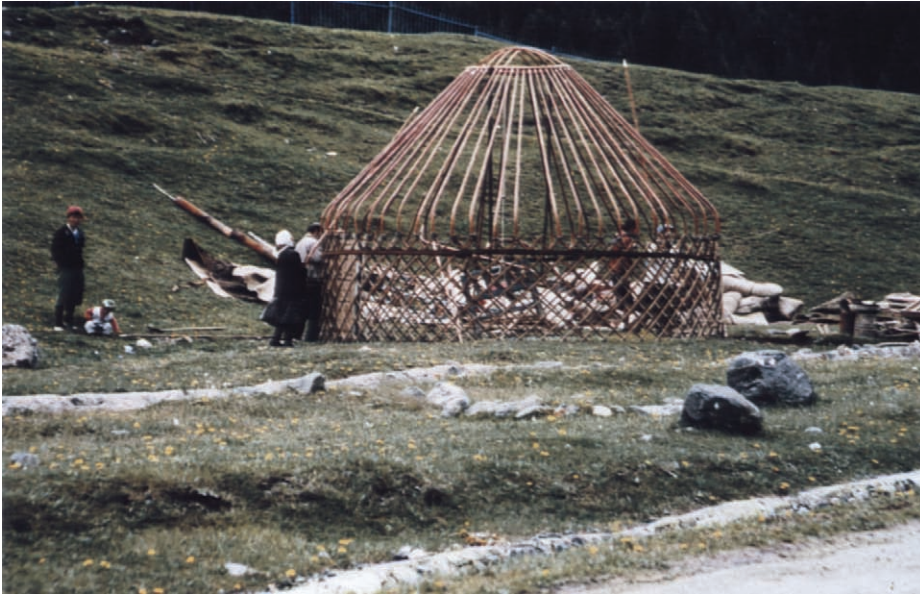
Figure 10. Erecting a framework for a ger , Xinjiang Uyghur Autonomous Region, June 1996. Photo: Emma C. Bunker
