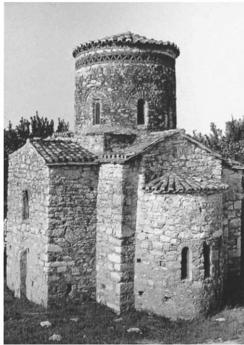
Figure 4. Church of Hagios Basileios tes Gephyras, near Arta, Greece (from the southeast). Second half of the 9th century (Photo: P. L. Vocotopoulos)
