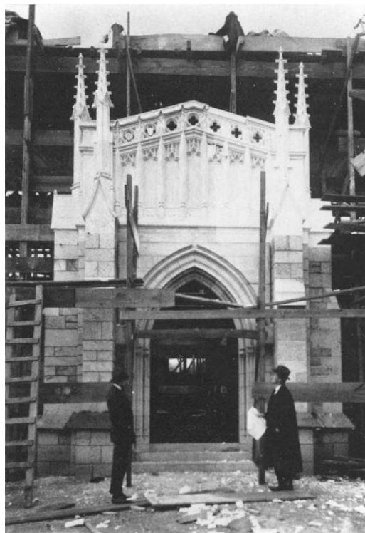
2. A full-scale plaster model of a gable in place on the south porch of the cathedral, viewed by Ralph Adams Cram and Raymond Pitcairn
