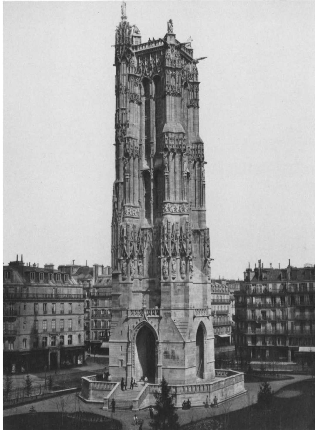
Fig. 80. Tour Saint-Jacques , ca. 1858. Albumen silver print from glass negative, 44.1 × 32.8 cm (17 3 / 8 × 12 7 / 8 in.). Canadian Centre for Architecture, Montreal
