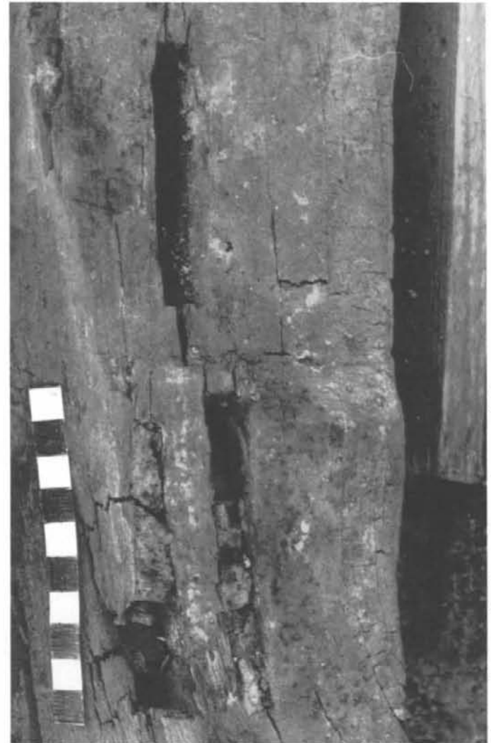
Pl. 116d. Detail of mortise-and-tenon joints.
