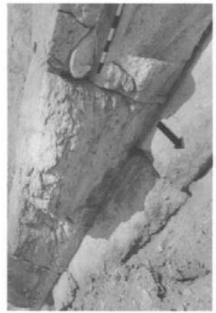
Pl. 8b. Remains of the casing blocks at the north side of pyramid I, with step for the false door.
