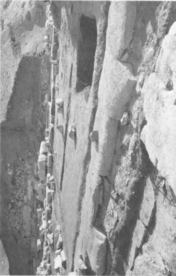
Pl. 42a. Foundations of the southern enclosure wall of pyramid 6 in the foreground, with shaft 14/8 to the right.
