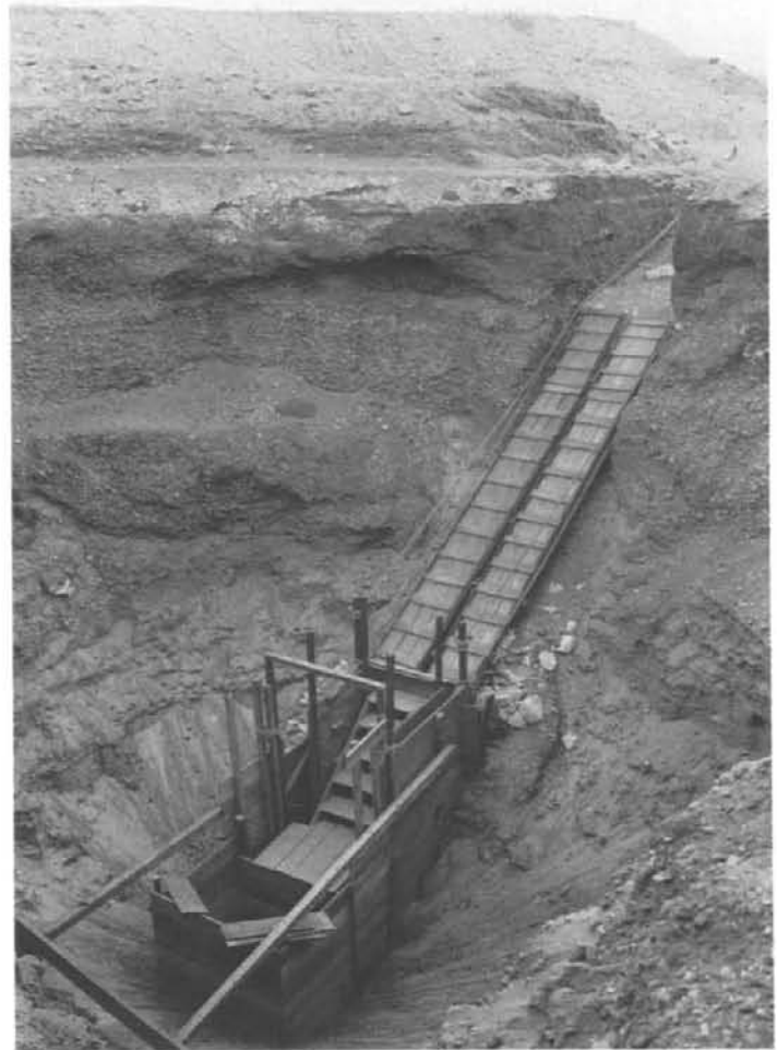
Pl. 36b. Excavation of shaft 2/14 using the caisson method during the 1931-32 season.
