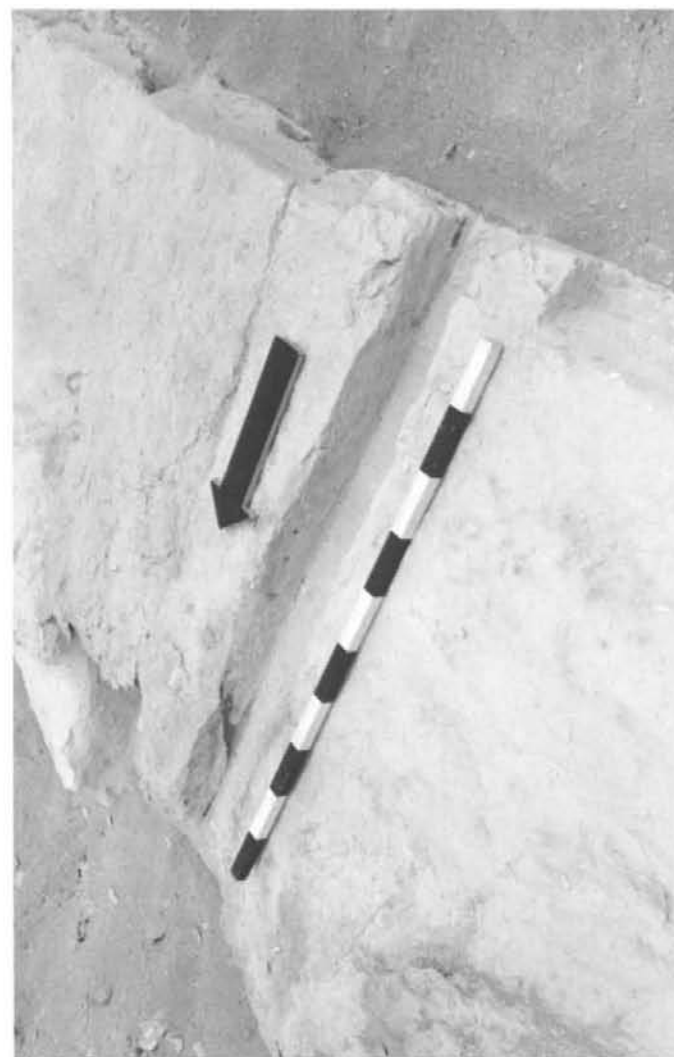
Pl. 31c. Drain in the southern enclosure wall of pyramid 4.
