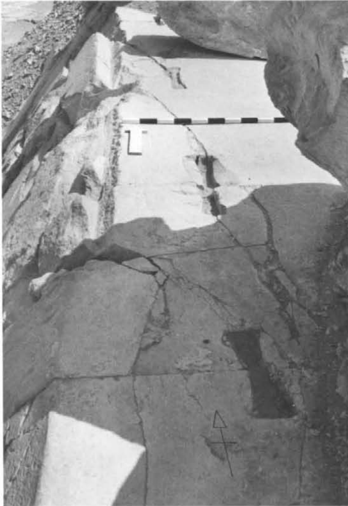
Pl. 112a. Cramps from the seventh course of the casing on the west side of the pyramid of Senwosret I (see cramp list p. 99, nos. 24–25).
