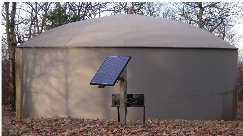
FIGURE 5.1 Small solar cell installation monitoring the water supply in Shenandoah National Park in Virginia.
