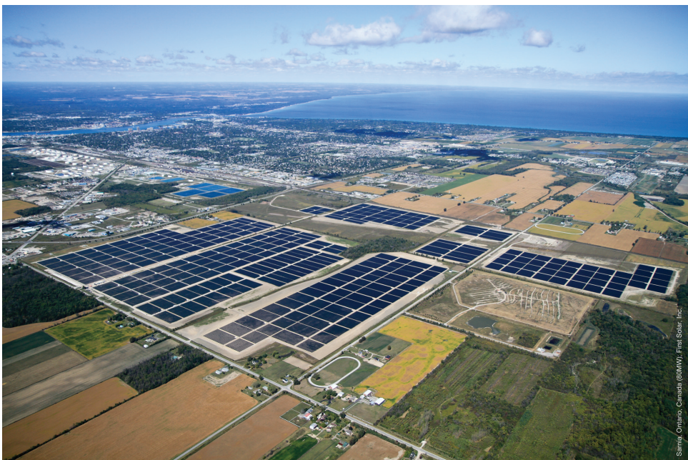
FIGURE 5.6 Eighty-megawatt thin-film cadmium telluride (CdTe)-based solar plant in Canada. SOURCE: Courtesy of First Solar.
